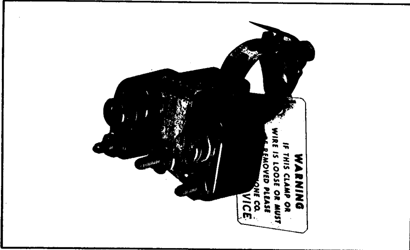
FIGURE 3. Front View of 123 Type Protector, 72A Bracket and Ground Clamp with Water Pipe Removed
