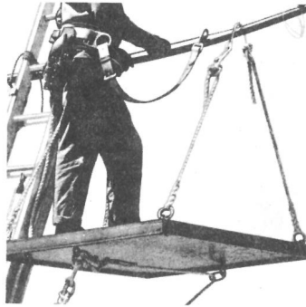
FIGURE 3. Method of Using Safety Strap When Working from Aerial Platform
